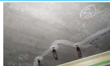
ひび割れ補修
